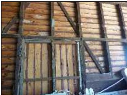
**Illustration 7: Interior of north wall showing framing and weatherboard construction.**
