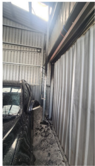
Heat damages to framing
