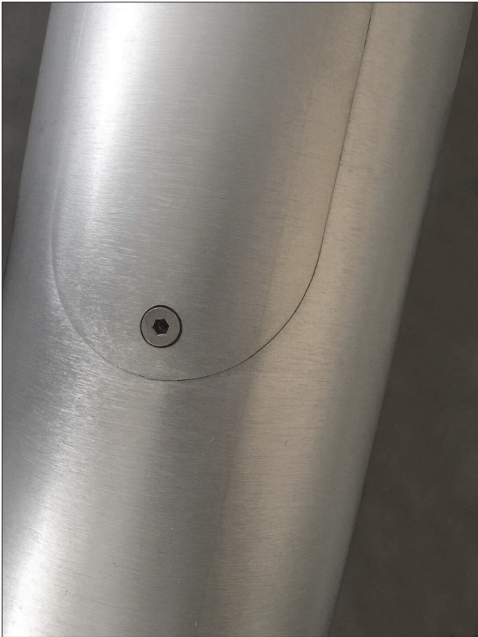
FLUSH HATCH DETAIL
