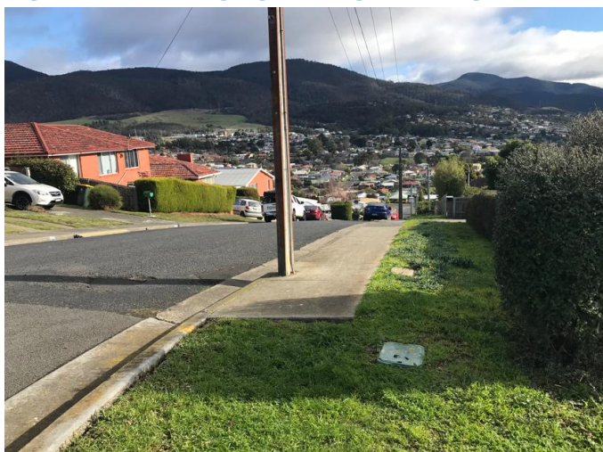
Figure 20 – Looking right along Thornleigh Street from proposed access.
