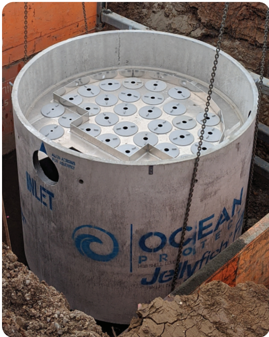
Figure 3: Jellyfish® precast manhole
