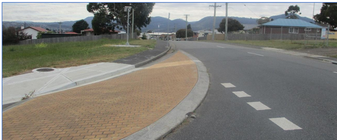
Photograph 6.4A – Available sight distance to the left
