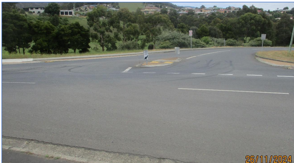
Photograph 6.3 – Junction of Allunga and Claremont Link Roads
